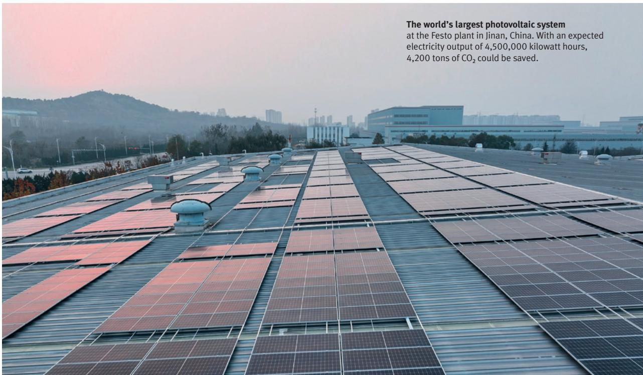
**The world's largest photovoltaic system** at the Festo plant in Jinan, China. With an expected electricity output of 4,500,000 kilowatt hours, 4,200 tons of CO<sub>2</sub> could be saved.
